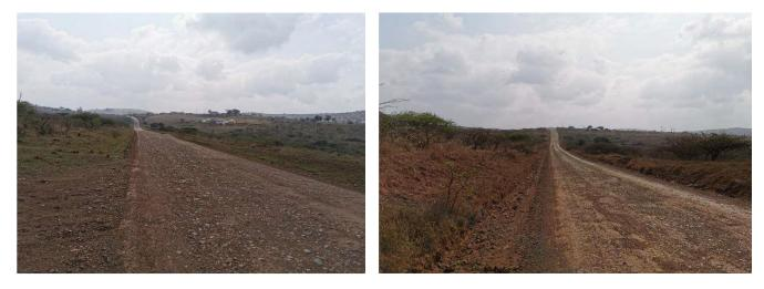
The objective of the project is to re-gravel of P494 from km 13 to 20 km. There is no gravel left on the current surface and is slippery when it rains the road requires new gravel surface layer to be placed.
